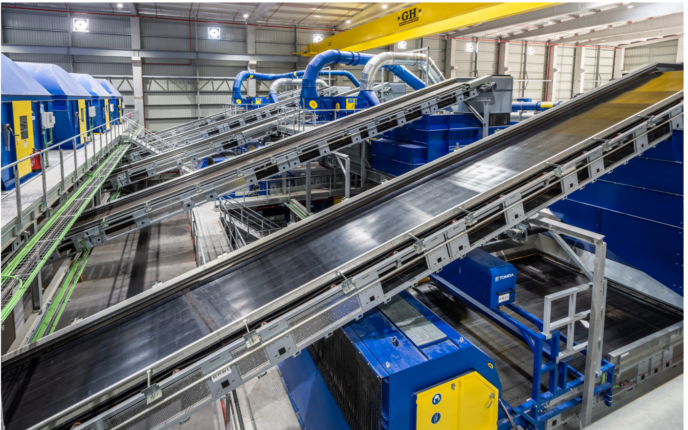
Each line in the new plant can select and pack more than 750,000 tons of recycled waste per year.
